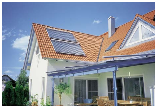
Figure 22 : High efficiency solar thermal vacuum collector systems; Source : Paradigma, Ritter Energie und Umwelttechnik, Karlsbad, Germany
