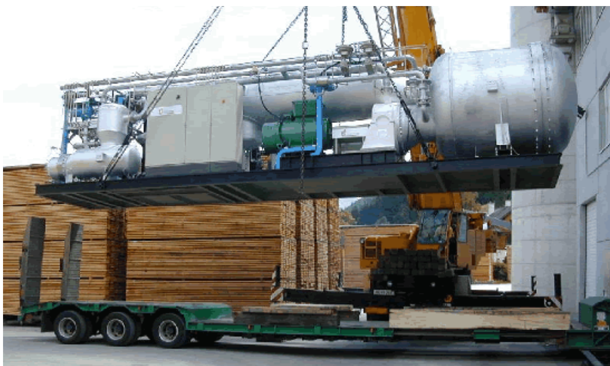
Figure 36 : An ORC power plant <88> ; Source :Turboden, Brescia, Italy.
